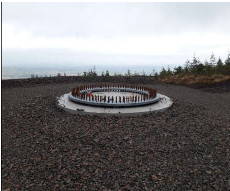
Plate 4-3 Finished Turbine Foundation
