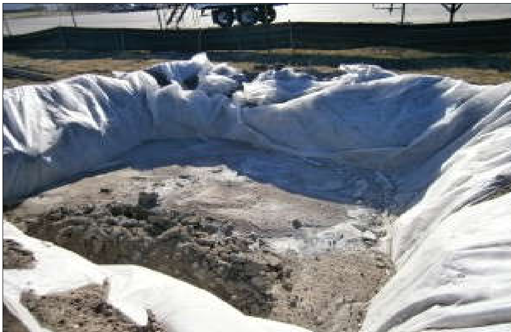
Plate 4-5 Concrete Wash Out Area
