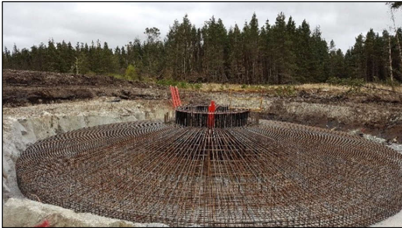
Plate 4-2 Turbine Foundation Anchor Cage surrounded by reinforcing steel.
