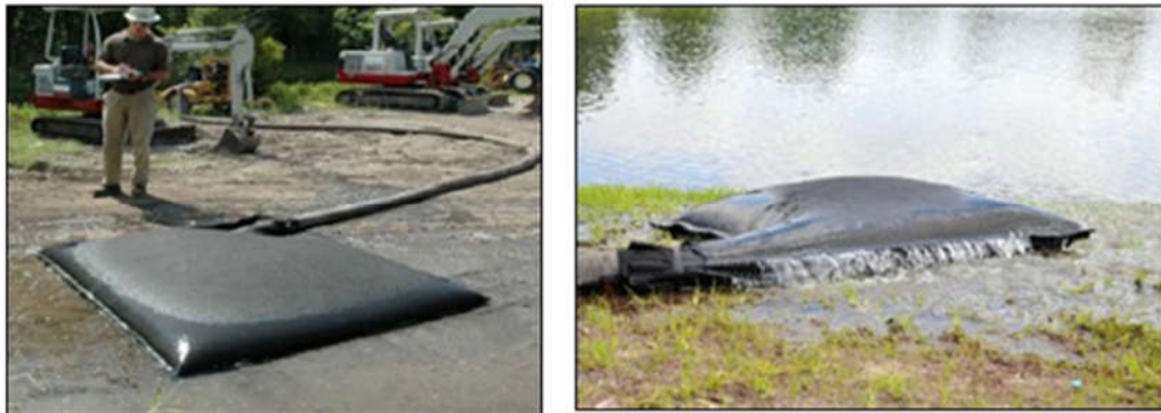
Plate 4-7 Silt Bag with water being pumped through.
