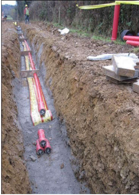
Plate 4-8 Typical Cable Trench View
