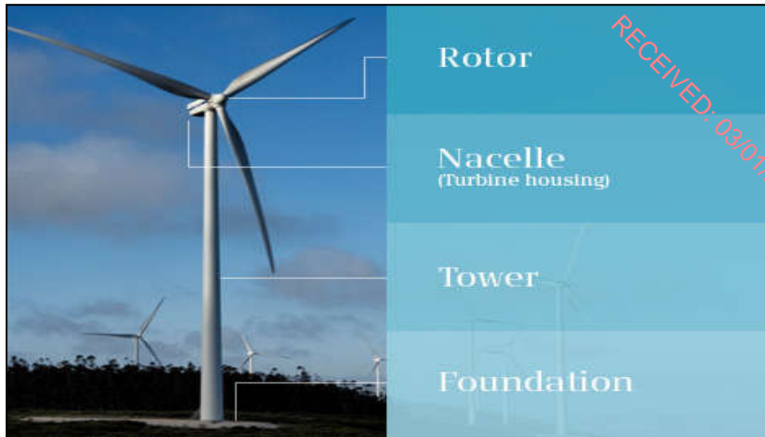
Plate 4-1 Wind Turbine Components
