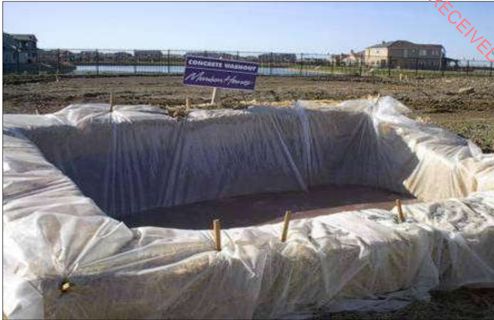
Plate 4-4 Concrete washout area
